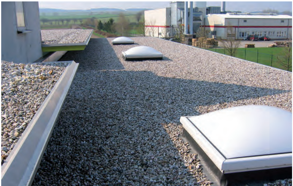
Flat roof with a gravel protection layer
